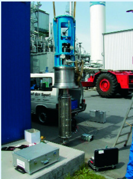
Last preparations of the sensors at the centrifugal pump before re-commissioning
